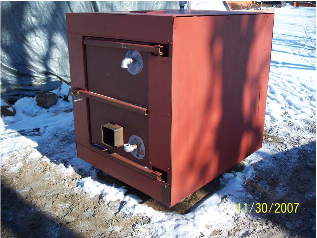
View of completed sheet metal installation to the stove housing front.
